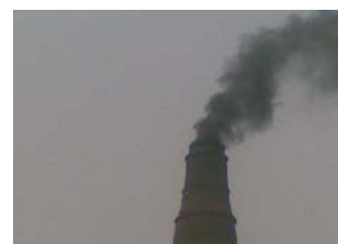
Dark smoke due to low quality coal and supplementary materials
